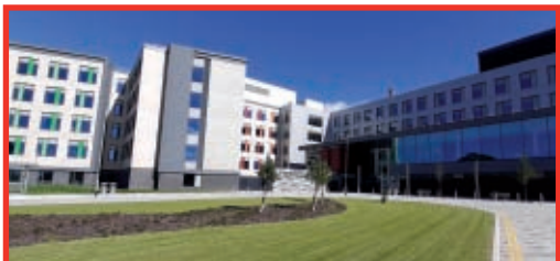
The new Grange University Hospital
