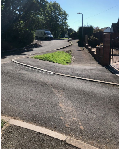
Photo 6: Informal A4042 Crossing – OHD
