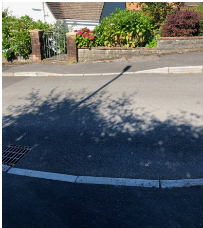
Photo 7: Informal A4042 Crossing – OHD
