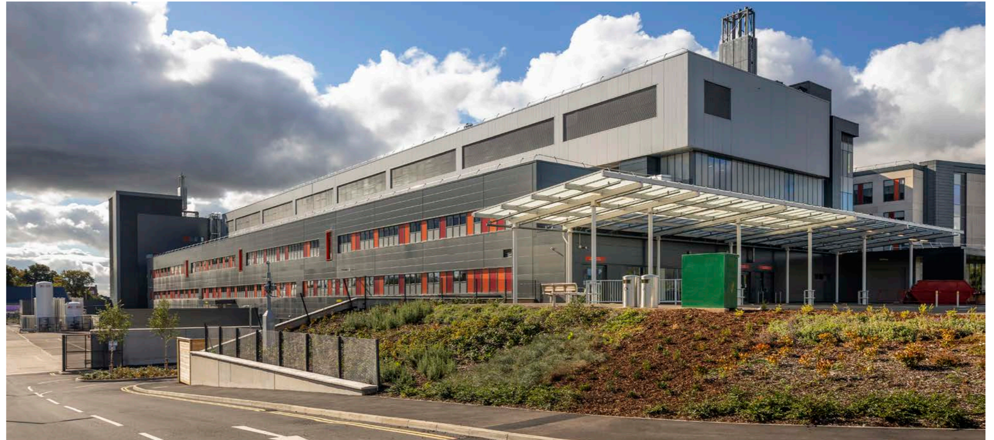
Location of the proposed extension in the foreground with Diagnostic & Treatment Block beyond
