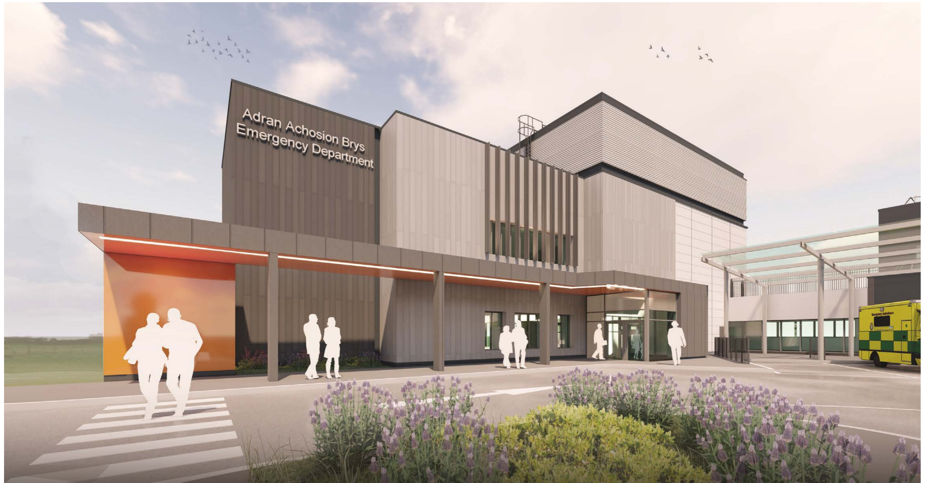
Final design visualisation of main entrance and canopy, with projecting entrance lobby facing the approach, screened from the adjacent ambulance bays and large format signage at high level.
