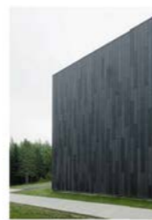
MAT 04: GRC rainscreen cladding
