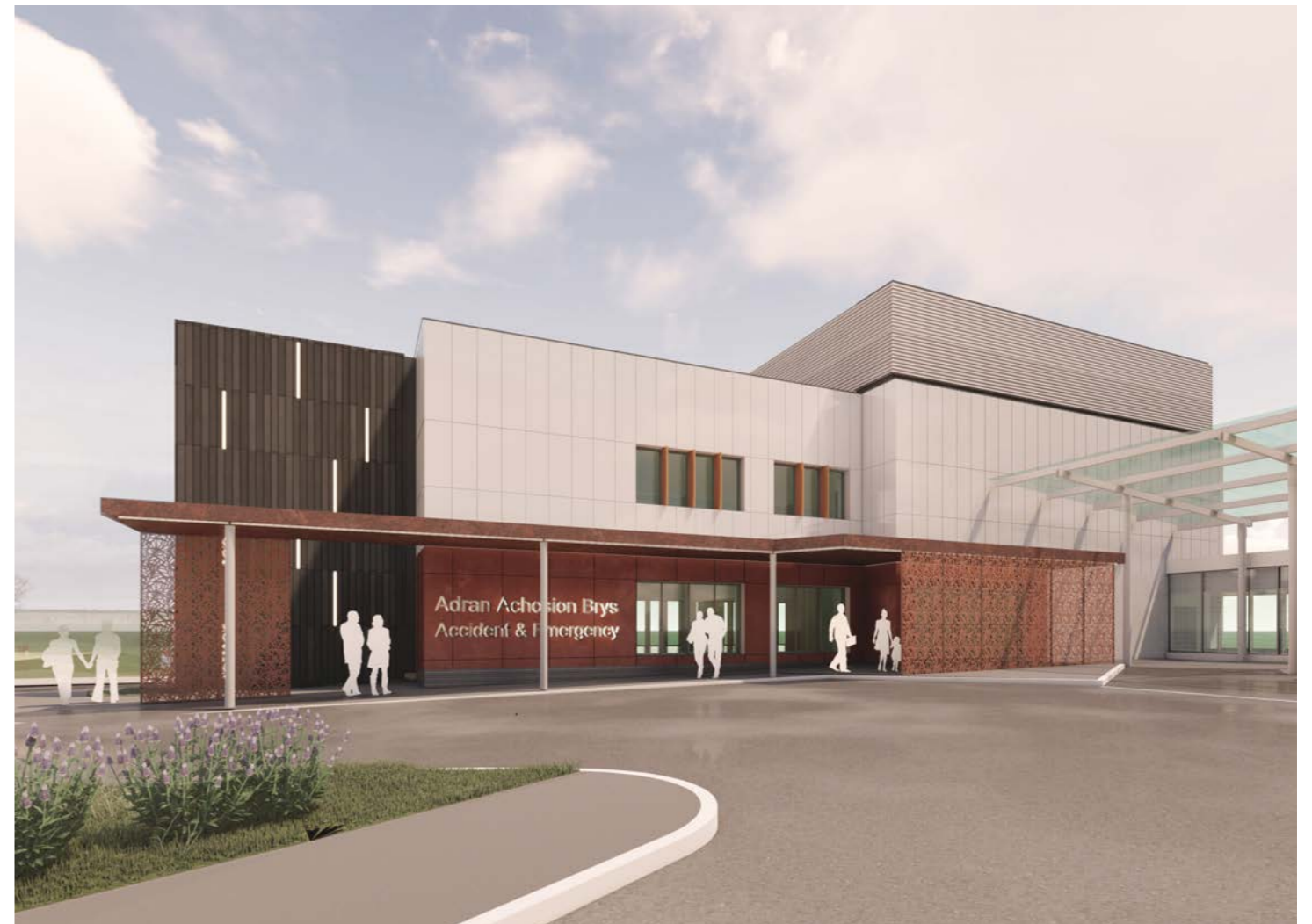
RIBA Stage 02 Visualisation indicating proposed extended canopy aiding legibility of entrance - February 2023
