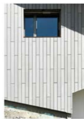
MAT02: GRC rainscreen cladding
