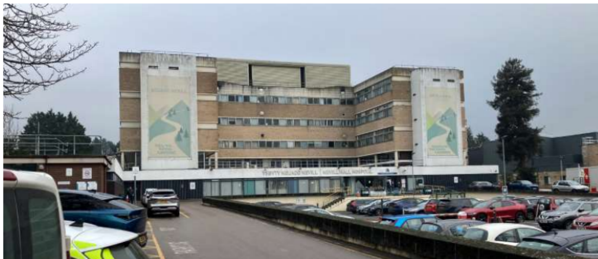
Figure 23: Picture of Nevill Hall H Block / Towers
