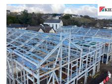
Heart Building works are also ongoing with the building now strapped to the main steel frame. The next phase of works is to remove the old roof and internal partitions and install a new steel support frame inside the structure, which will ultimately carry the new roof.
